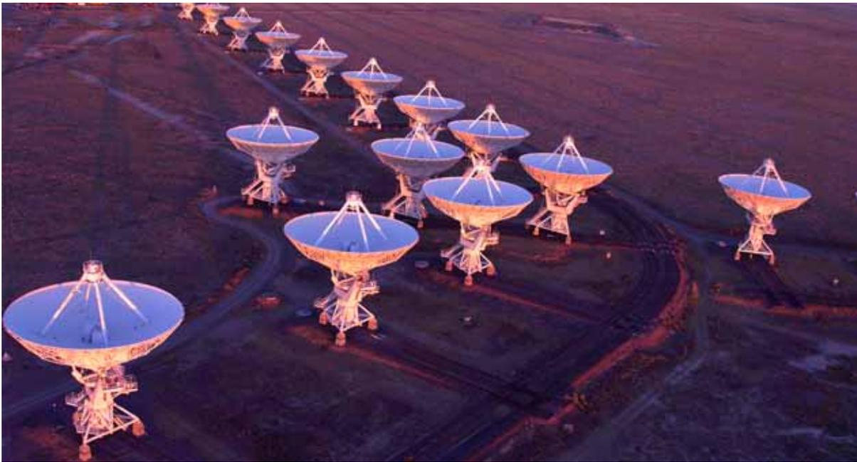
**Figure 2.** The National Radio Astronomy Observatory Very Large Array. Each radio telescope of the 27-element interferometer has a diameter of 82 feet. Each telescope can be moved with a special transporter.
